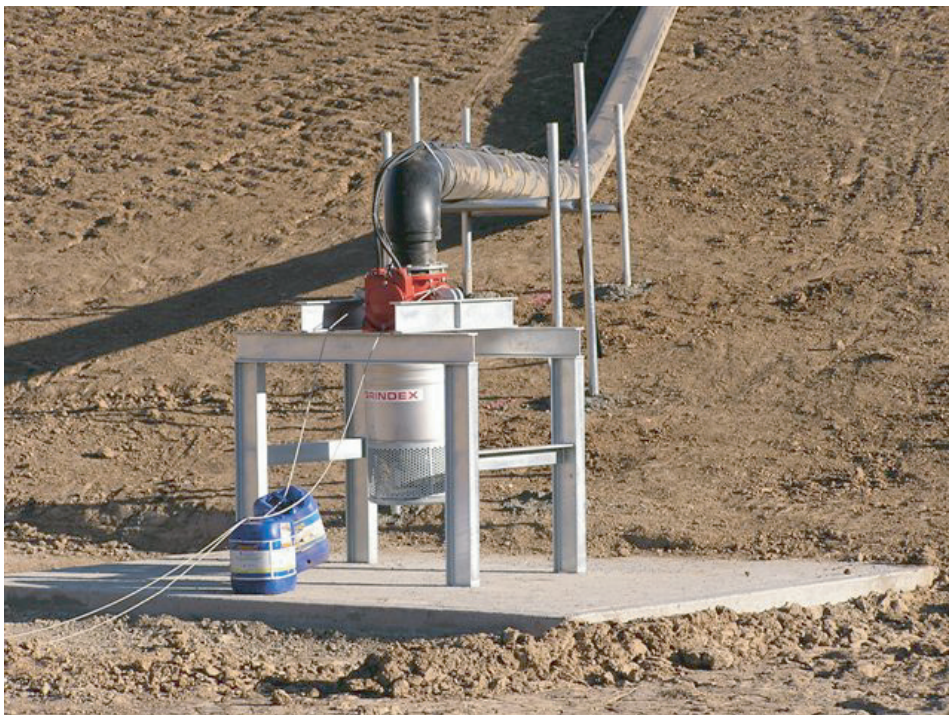
The Grindex Maxi pump and discharge hose are mounted to steel frames. The floats are attached to the pump using stainless steel wire and are used to locate the pump for bringing to the surface.
